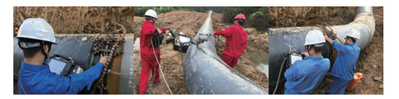
Crawler CPS-01 for long-distance oil and gas pipeline.
